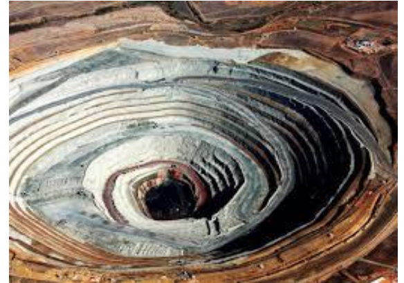
Mining Machine Control
